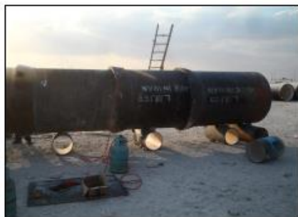
View on DN1400 Bell & Spigot pipe joint
