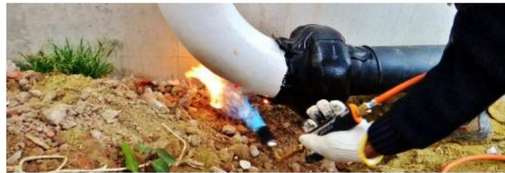
Both FCWS-F as installed on DN150 flanges.
