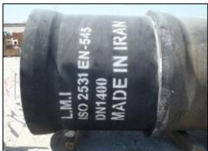
View on DN1400 Bell & Spigot pipe joint
