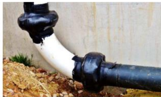
Both FCWS-F as installed on DN150 flanges.
