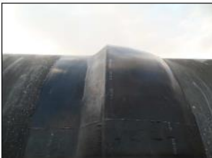
View on DN1400 Bell & Spigot pipe joint
