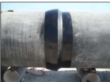
View on DN1400 Bell & Spigot pipe joint
